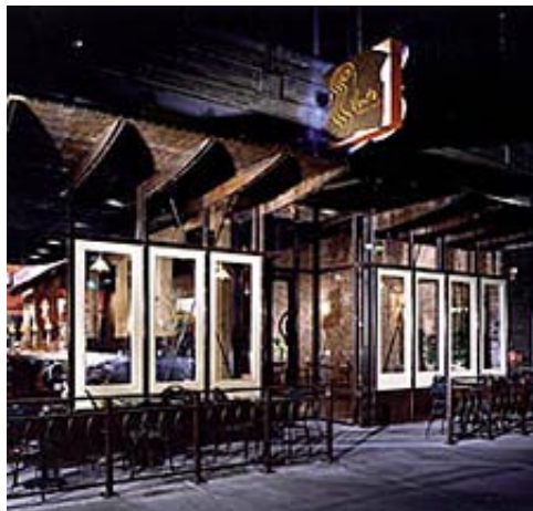
The exterior of Vesta Dipping Grill features a custom-fabricated steel-and-glass storefront, designed by Roth Sheppard Architects and constructed by Goog Custom Design.
